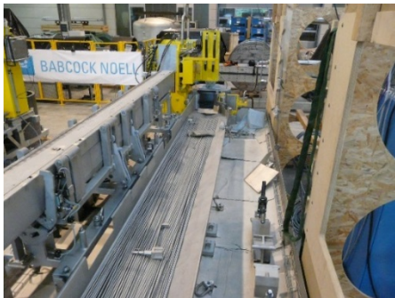
Fig. 1 Overview: Waste dismantling, long rods
