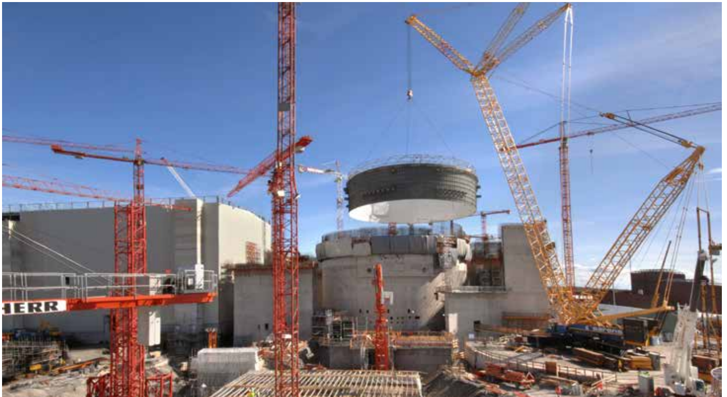
Olkiluoto 3: Lifting of the second liner ring
