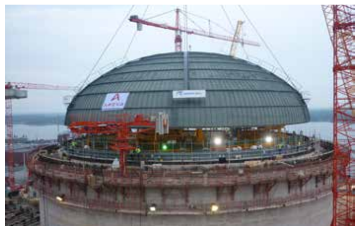
Olkiluoto 3: Lifting of the dome
