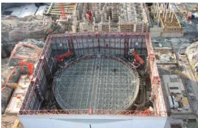
Olkiluoto 3: View into the reactor building after positioning of the cup
