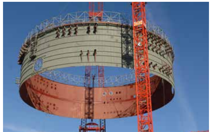
Olkiluoto 3: Lifting of the first liner ring
