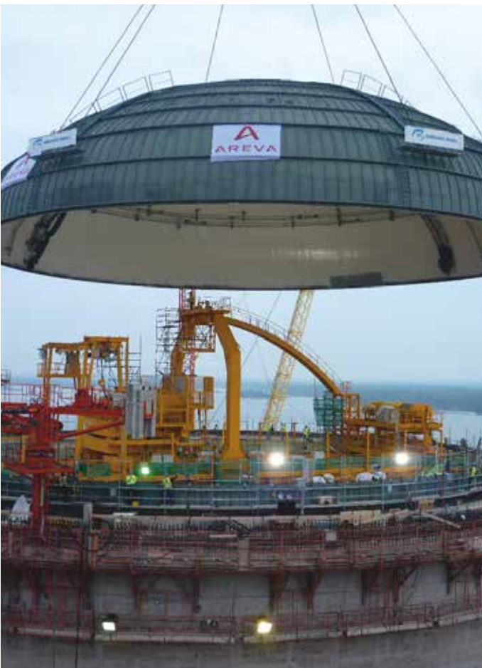
Olkiluoto 3: Lifting of the Dome
