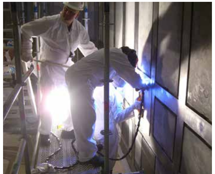
Olkiluoto 3: Pool Liner - Welding of Liner Sheets
